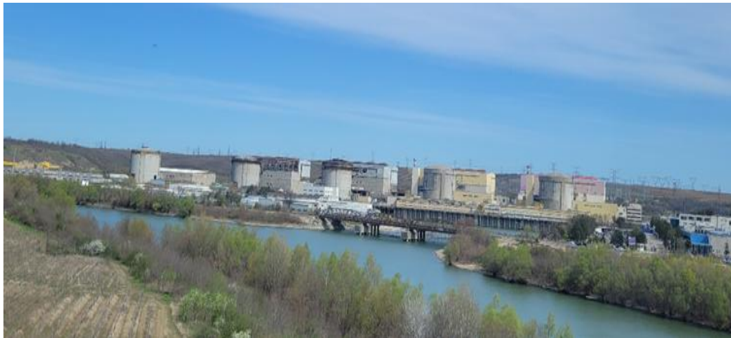
Fig. 1. View of the Cernavoda Nuclear Power Plant site.
